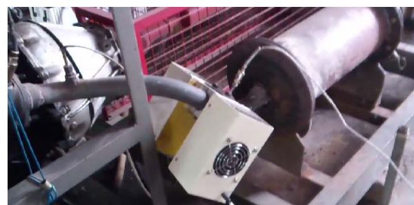
Fig. 9: Assembly and Installation of a TEG
